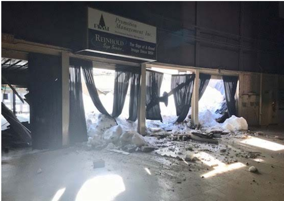
Nearly 6 feet of snow fell into the inner lobby of the Brown County Veterans Memorial Arena on April 20 when a record snowstorm pounded Green Bay, Wis. (Photo: Terry Charles / PMI Management Group)
